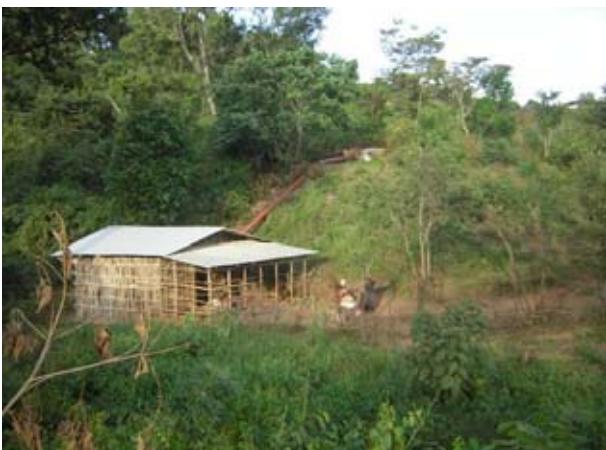
Grinding mill house with penstock and would fit with the forebay/water reservoir as a logical sequence. By Dirk Hillerkus, 2009.
